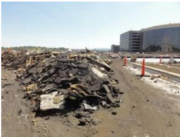
Tear off pile.
