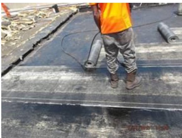
Temporary roof installation
